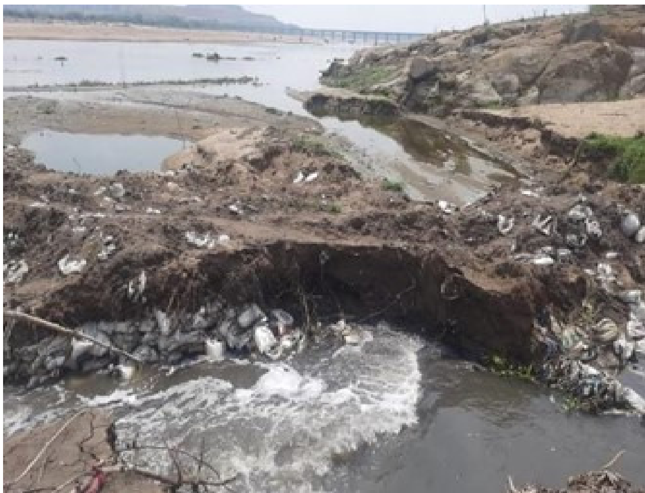
Figure 9: Wastewater discharge without treatment
