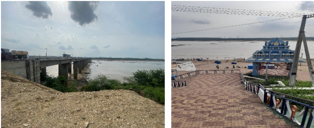
Figure 42: Bhadrachalam Bridge on Godavari river and Bhadrachalam Temple Ghat
